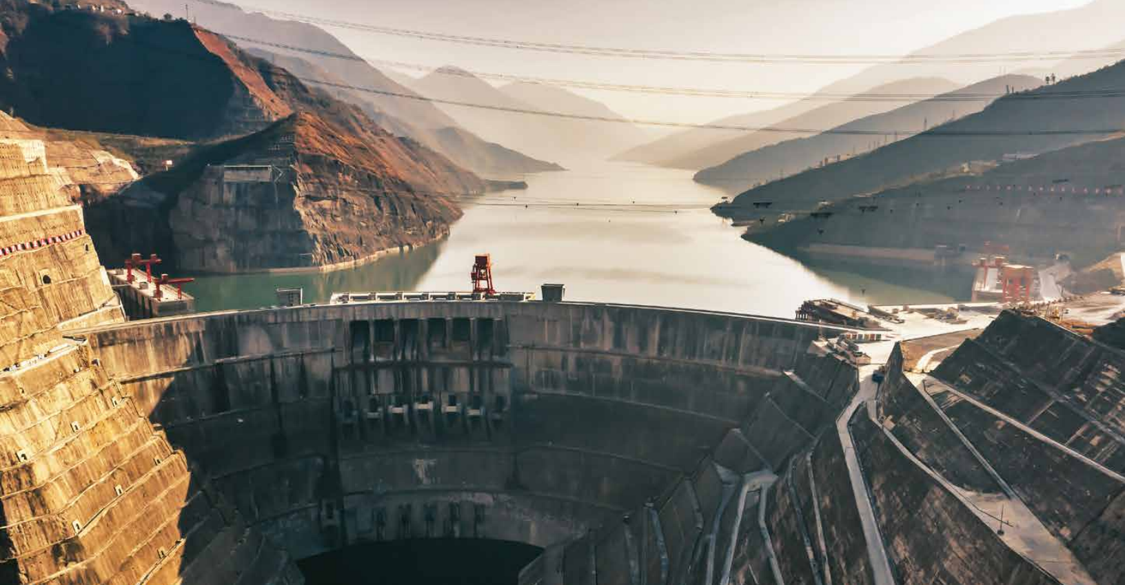
At left, a solar farm in Qinghai province, and, above, the Baihetan hydropower station.
