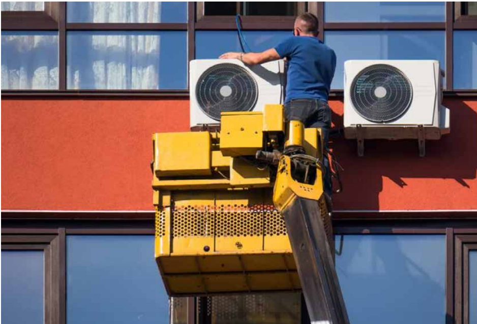
Installing a heat pump.
