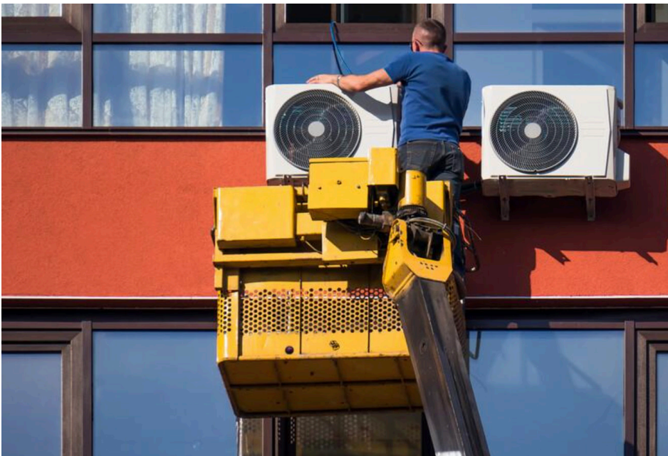
Installing a heat pump.
