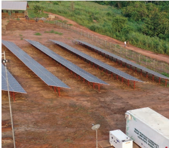
The Mokoloki minigrid is powered by solar panels, lead-acid batteries, and a supplementary diesel generator.
