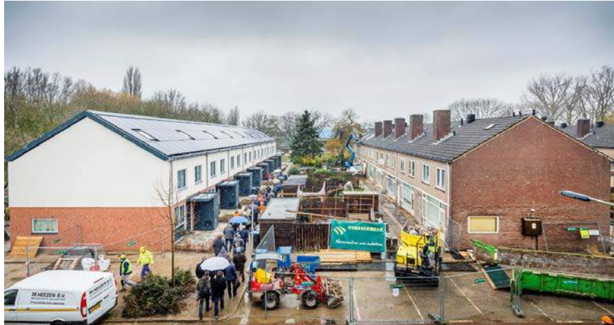
Figure 2. Typical row house typology in the Netherlands before (right side) and after (left side) retrofit
