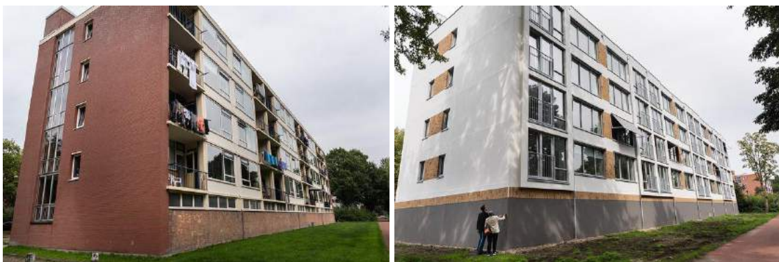
Figure 1. Energiesprong project before (left) and after (right) renovation
