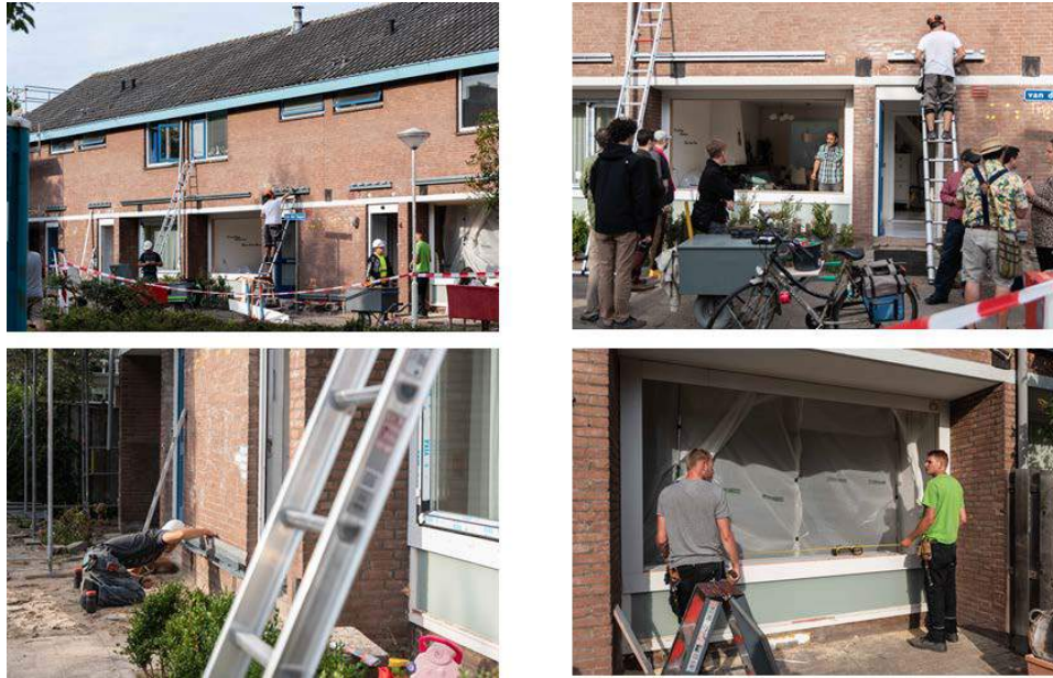
Figure 8. Installation process images for RC Panels
