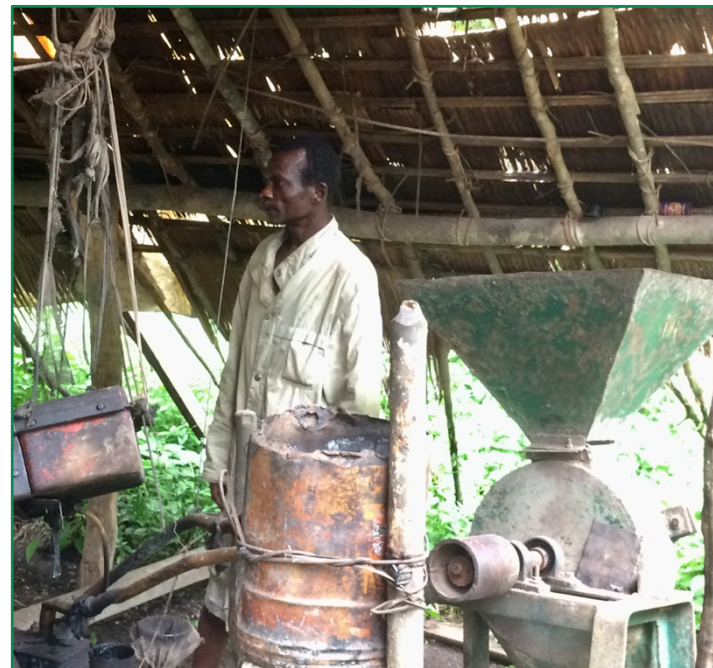
Local farmers use diesel generators to run machines that process palm oil, cassava/gari, and other crops
