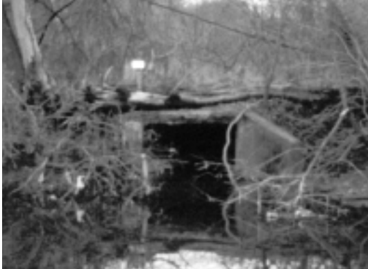
A combined sewer overflow structure along Nine Mile Run.
