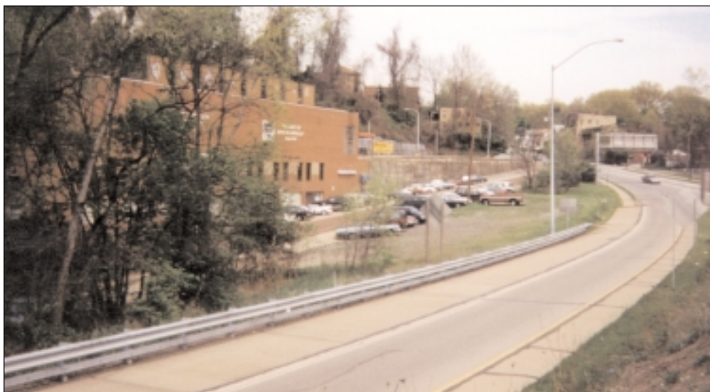
The parkway ramp and the underutilized commercial building at the Regent Square Gateway site. Old Braddock Avenue runs alongside the building and terminates at the Wilksburg Culvert outfall hidden in the trees to the left. Photograph by Richard Pinkham, RMI.
