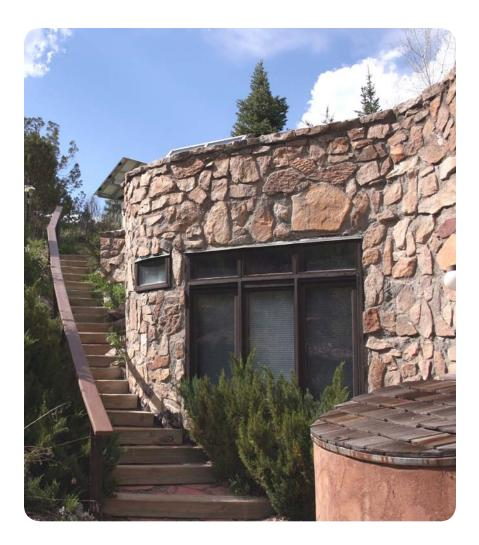
**West Bedroom:** The bedroom wing, being far from the greenhouse (the "furnace" of the building), is heated by its south- and southeast-facing windows (plus surplus heat from the people, lights, and minor heat leakage from a superinsulated solar-hot-water storage tank), so it stays a few Fahrenheit degrees cooler than the main wing, yielding more comfortable sleeping conditions.
