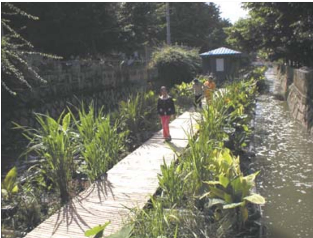
Baima Canal, essentially an open sewer for 12,000 people in Fuzhou, China. In 2002, Ocean Arks International ( www.oceanarks.org ) installed a bioremediation system that uses floating rafts of plants, microorganisms and aquatic life, combined with an aeration system. Drawing upon natural technologies found in ponds, marshes and streams, the system has dramatically improved canal water quality.
