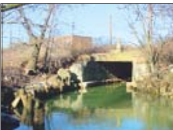
Before and after: Daylighting Kingsbury Run
