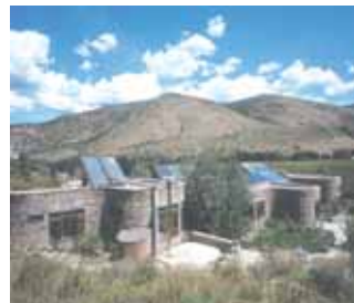
RMI's super efficient headquarters building located in Snowmass, Colorado.
