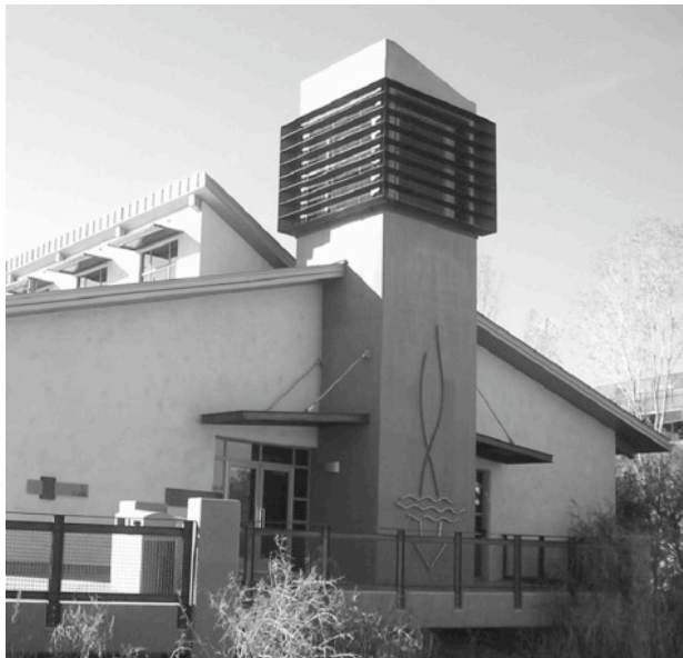
Figure 8: This downdraft cooling tower and pictorial diagram demonstrate a green building strategy and facilitate the visitor's experiential learning. Credit: Erik Bonnett.
