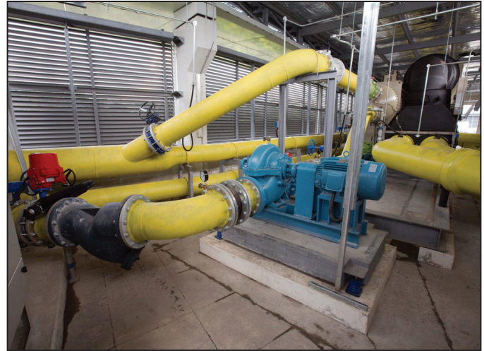
Figure 7: A Factor Ten design by Eng Lock Lee, with larger-diameter pipes and smooth transitions instead of right-angle bends.
