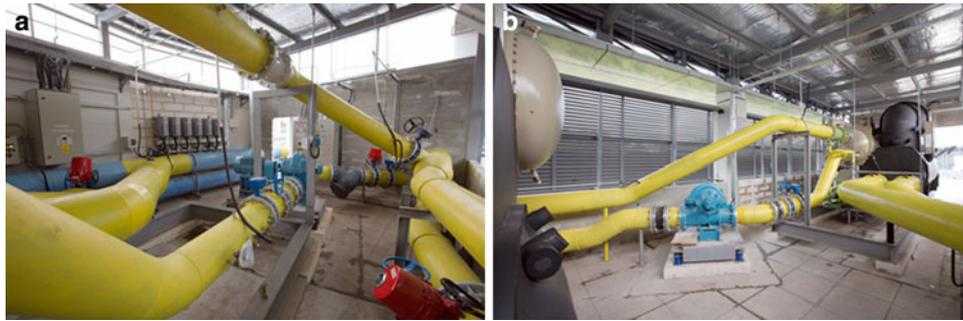
**Fig. 4** Cooling-system supply piping for a Singapore biotechnology facility, designed by LEE Eng Lock. The creative layout (vertically stacked to save costly space), direct diagonal runs, and Y- and “sweet” bends reduce friction 69% compared with normal orthogonal
