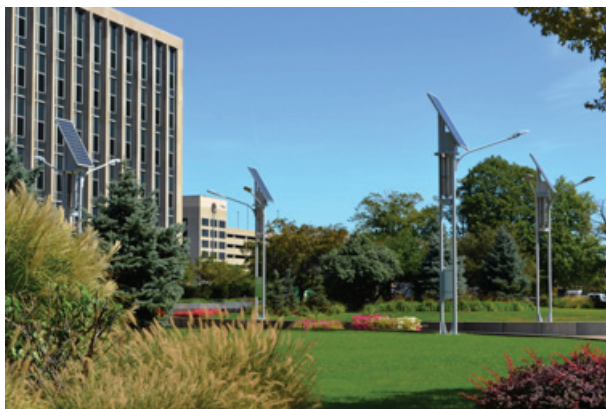
The Indianapolis City-County Building post-retrofit.
