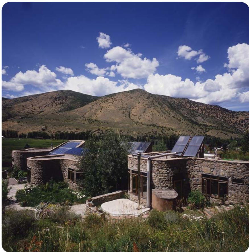
and partly for backup heating. The passive solar design also incorporates daylighting and natural ventilation while preserving viewlines and minimizing noise.
