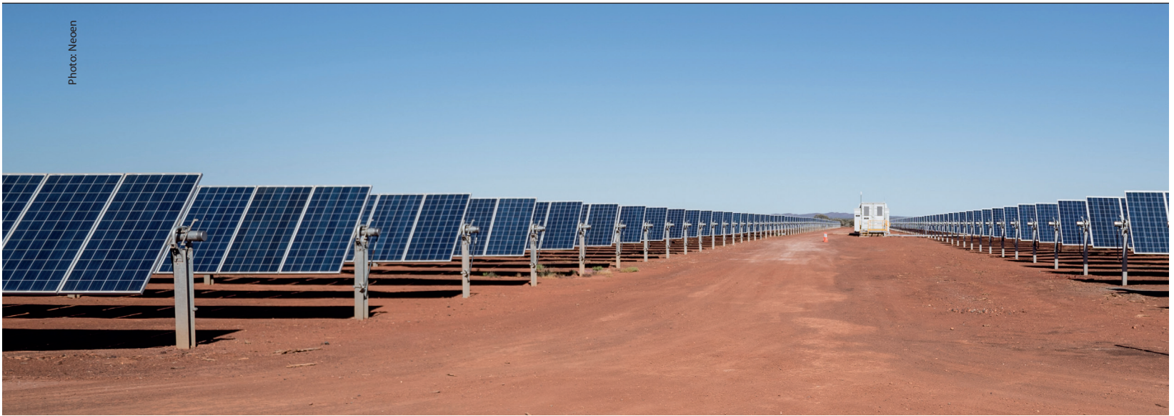
The 10.6 MW solar and 6 MW storage system at the DeGrussa gold-copper mine in Western Australia is the largest off-grid solar and storage system powering a mining site. The system was developed by Neoen for the mine owner, Sandfire Resources.
