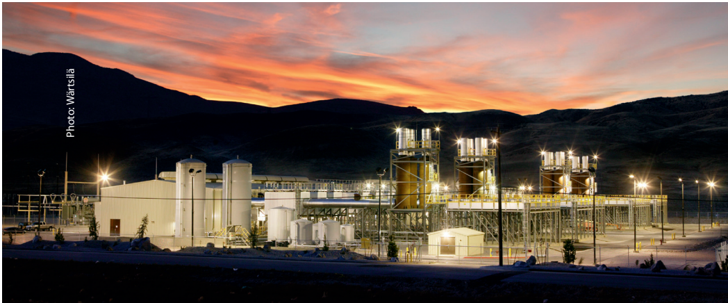
The Barrick gold mine in McCarren, Nevada, has a 1.5 MW solar system, in addition to a 116 MW gas power plant supplied by Wartsilä.
