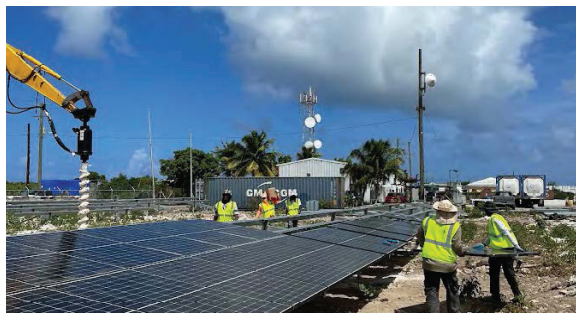
Construction of the first ground-mount solar project on Anegada British Virgin Islands, where it will supply the majority of generation for the utility.
