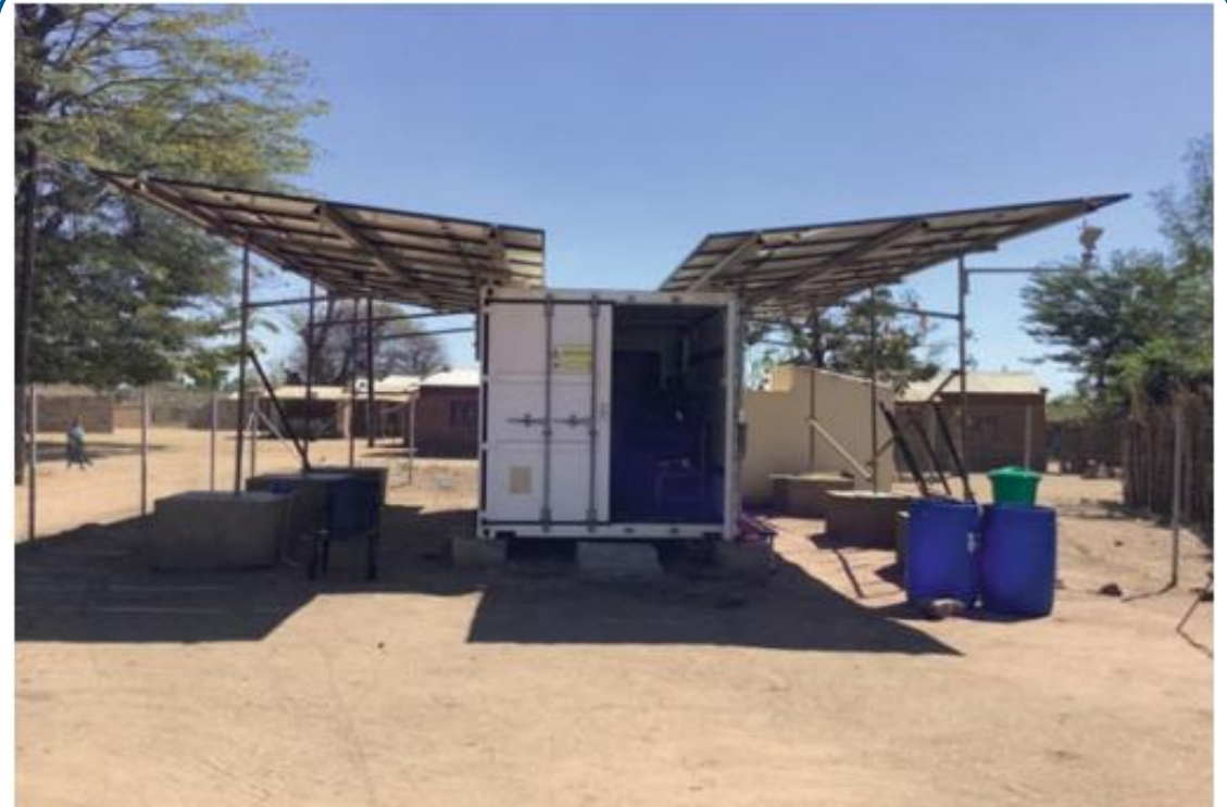
A climate-resilient Mthembanji solar PV minigrid in Malawi
