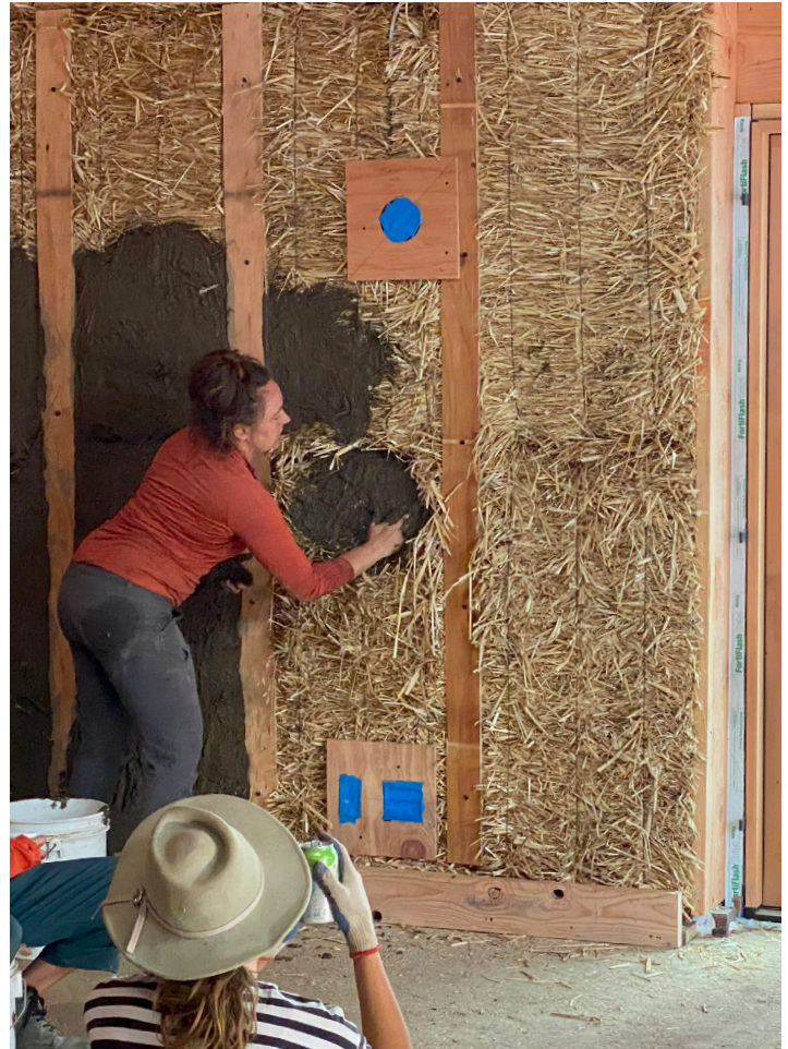
Application of earthen plaster over strawbale insulation
