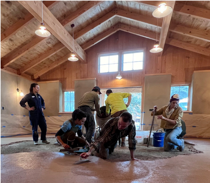
Installation of the finish coat of the earthen floor
