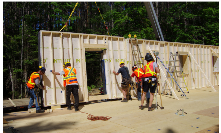
Installation of prefabricated wall panels
