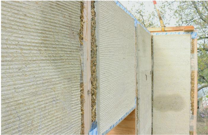
New Frameworks Panels being installed for the Terra 600 walls. The straw in these panels stores over 6,000 kg of CO<sub>2</sub>e! The panels are easily installed using a telehandler, and can be moved around on site easily to facilitate installation.
