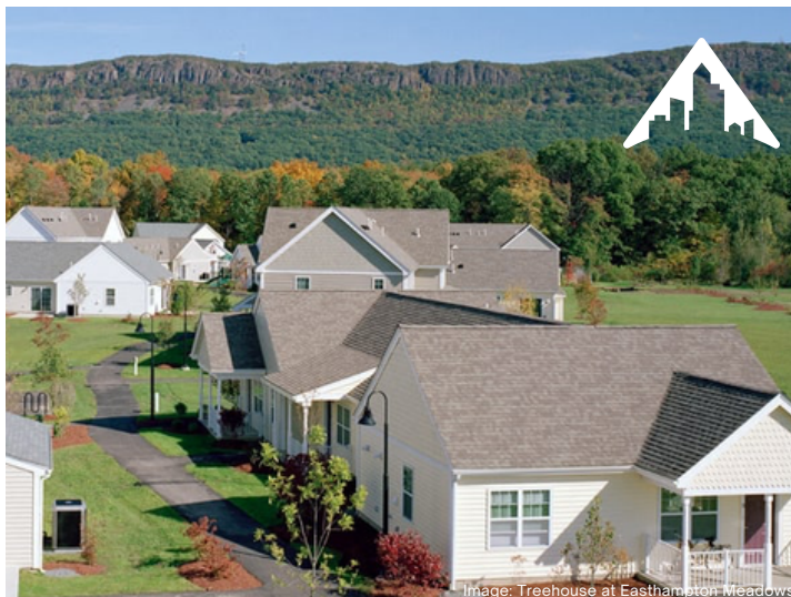
Treehouse at Easthampton Meadows, prior to renovations.
