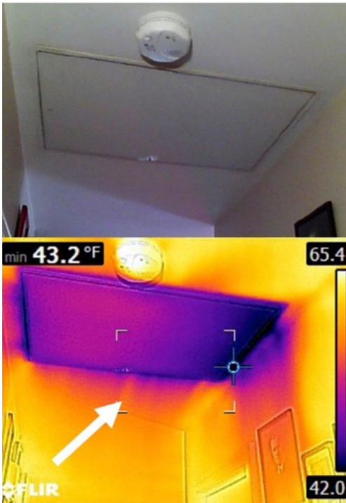
Thermal bridging and air leakage shown at attic hatch without gasket (left) and areas around windows (right).
