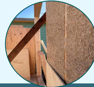
Prefabricated straw wall panels
