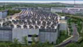
Data center in Ashburn, VA
