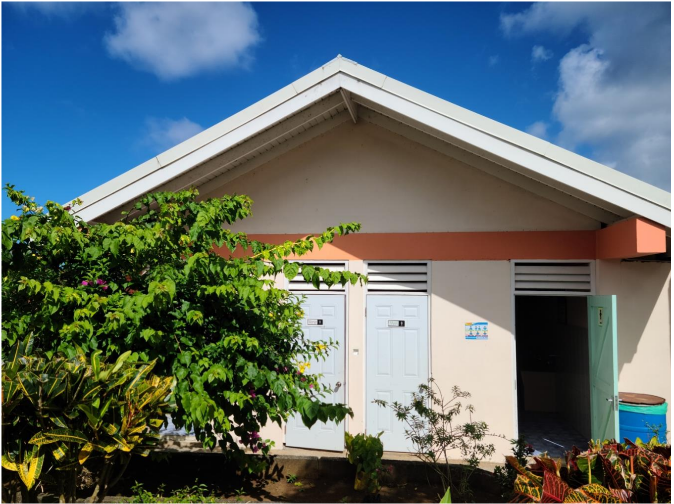
Figure 1-4: Paix Bouche Primary School, Bathroom Building
