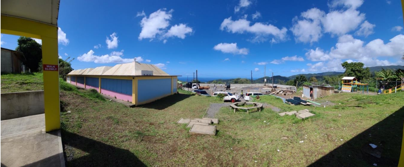
Figure 1-2: Morne Prosper Primary School, Old Building
