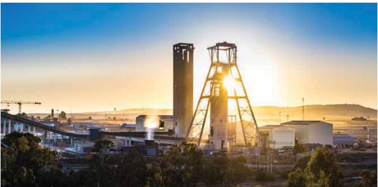
Twin Shafts at South Deep, South Africa
