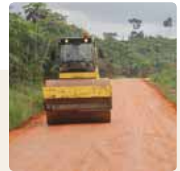
Road repair near Tarkwa
