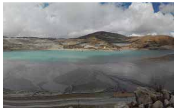
Tailings storage facility at Cerro Corona, Peru
