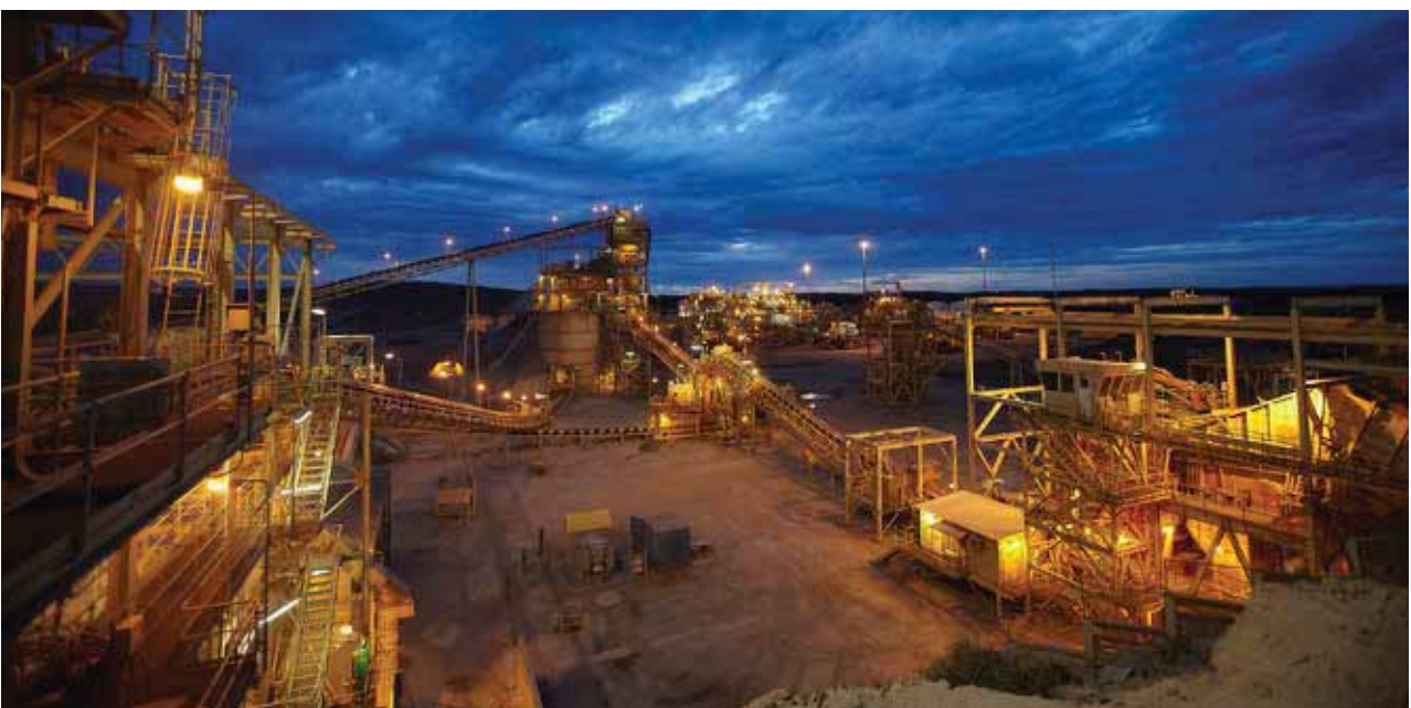
Processing plant at Granny Smith, Australia
