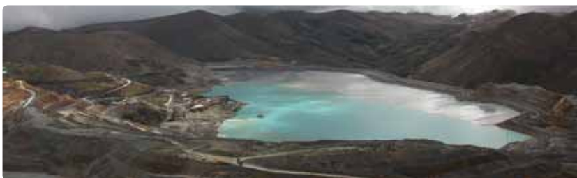
Cerro Corona tailings storage facility
