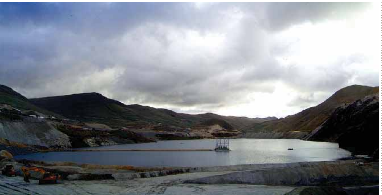
Tailings Storage Facility at Cerro Corona, Peru
